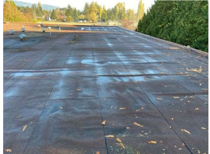
Photo 21: Widespread blisters, ridges and worn membrane on Building B roof.
