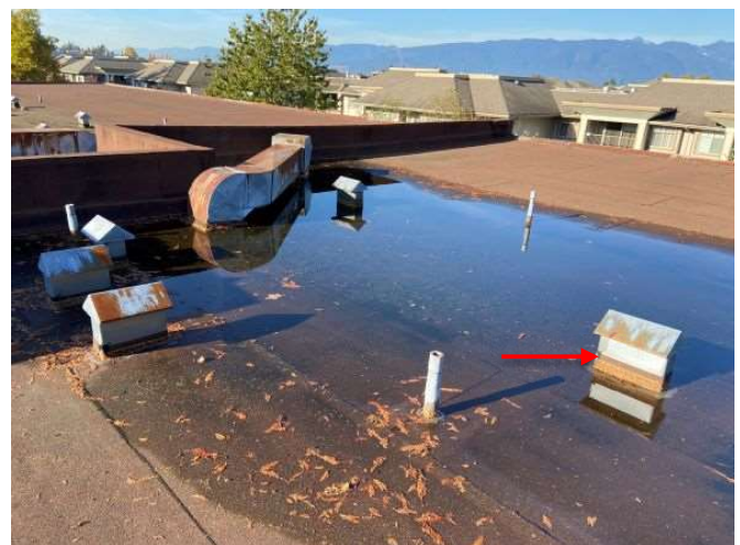
Photo 23: Extreme ponding water on Building A roof. Note that water level has dropped 3" from max height.
