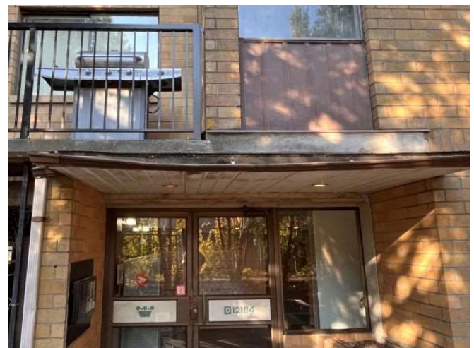
Photo 26: Sagging eave at Building D canopy.
