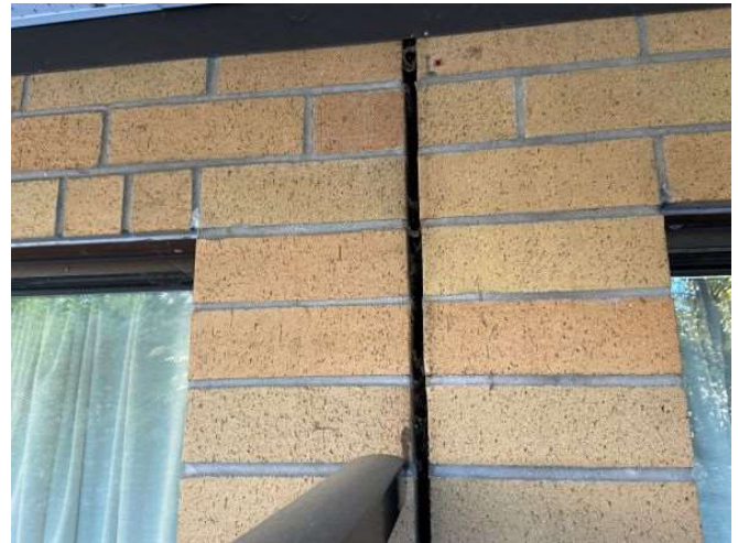
Photo 16: Unsealed masonry control joint.
