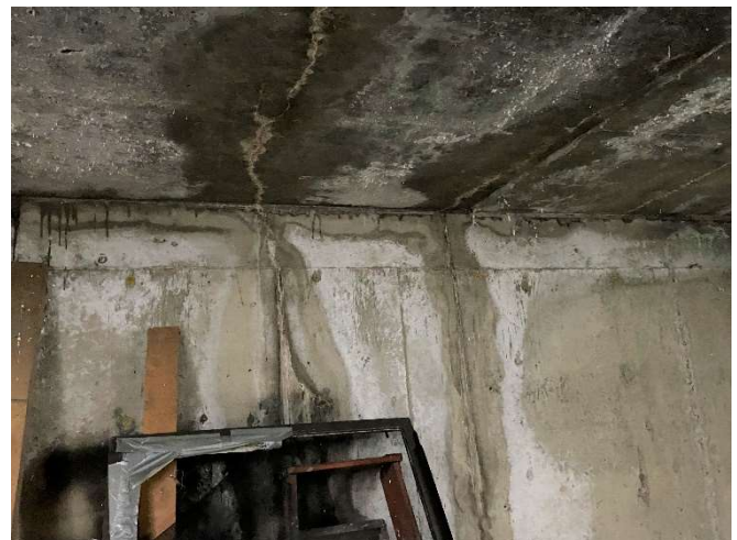
Photo 9: Active water leakage through roof deck at Building A maintenance space
