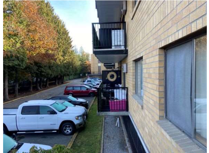
Photo 2: Typical balconies including concrete slab at the 2 nd floor and wood structures on the 3 rd and 4 th floors.
