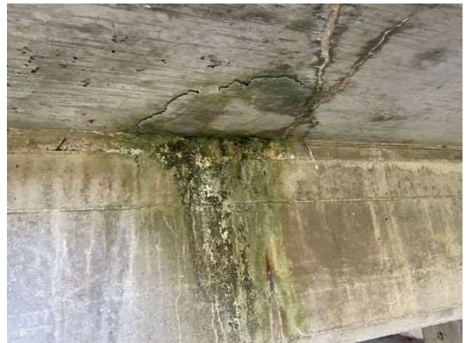
Photo 6: Leaking crack and spalled concrete on 2 nd floor slab soffit, south elevation of Building C.
