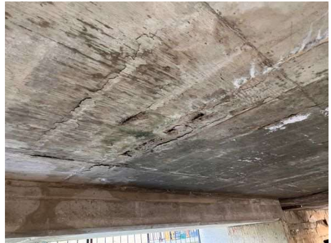
Photo 10: Building B – Soffit delamination and spalling.
