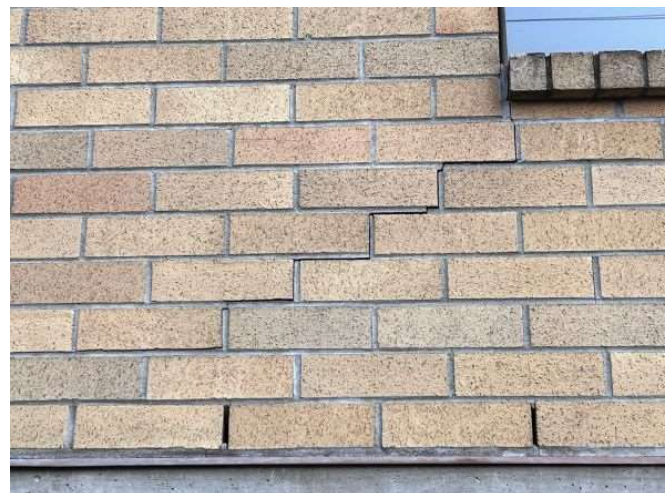
Photo 14: Step cracking at window opening.
