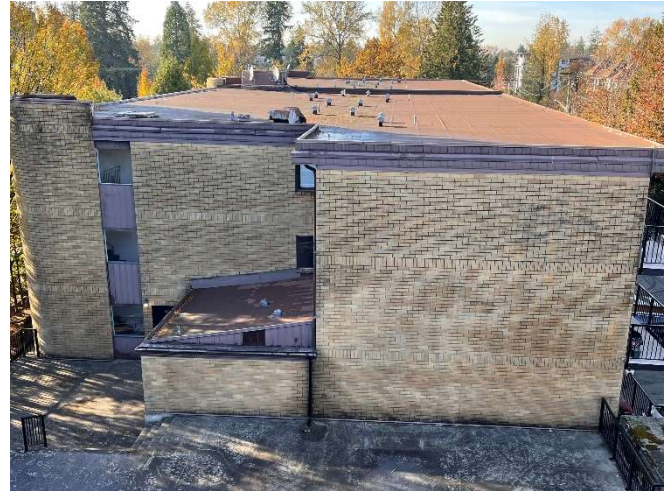
Photo 13: Typical exterior masonry clad walls.
