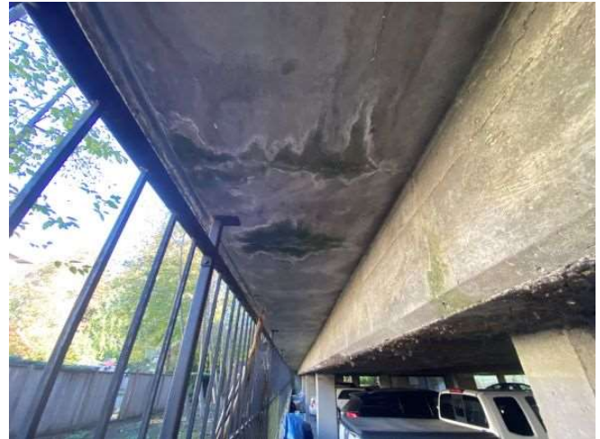
Photo 5: Leaking cracks in balcony slab, north elevation of Building A.
