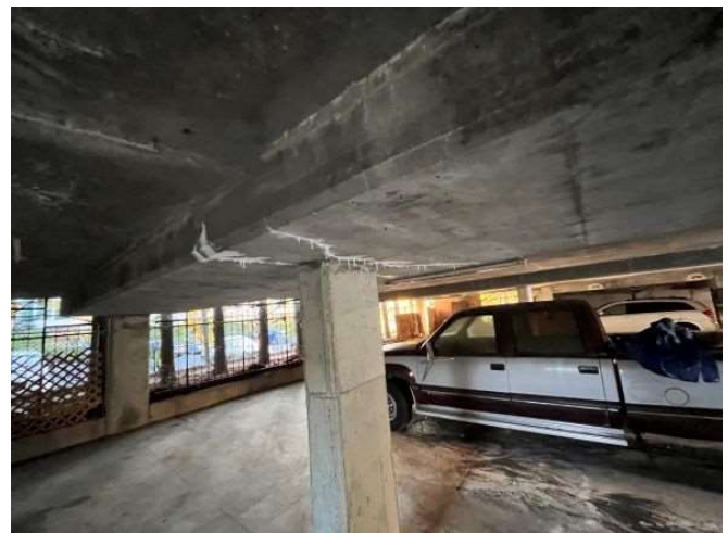
Photo 11: Buildings C/D – Active water leakage.
