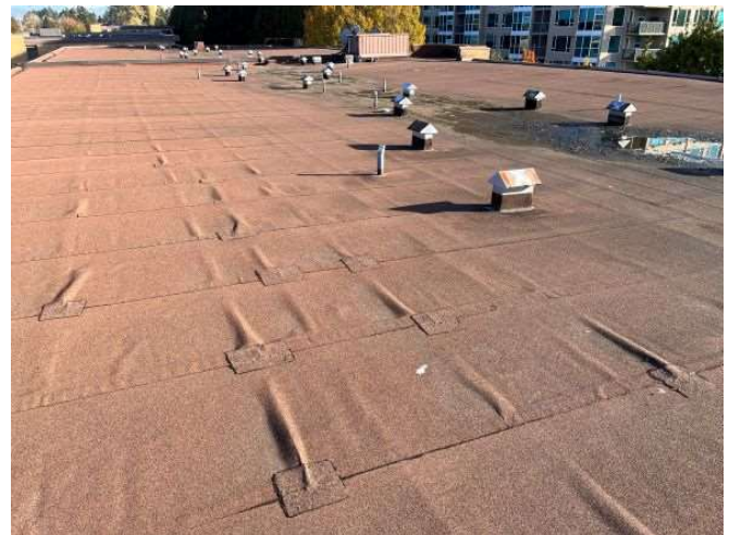
Photo 22: Patches at ridges on Building D.
