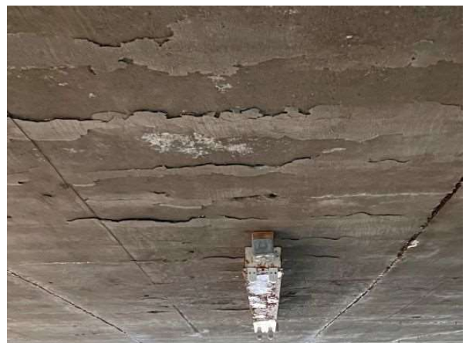
Photo 12: Building A maintenance space - Active water leakage through roof deck and spalling concrete.
