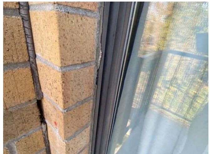
Photo 17: Poor sealant application at door jamb and no sealant at control joint.
