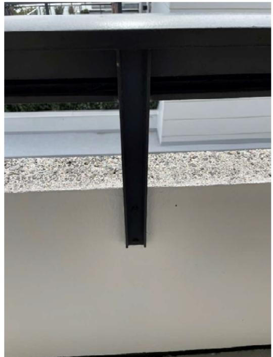
Photo 20 - Balcony guardrail connection.
