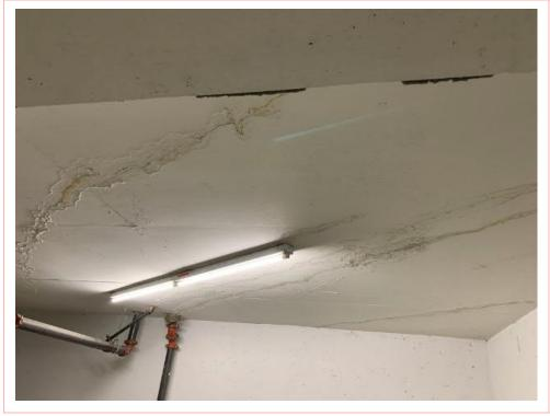
Photo 22: Evidence of leakage on soffit at northwest corner of P3-level.
