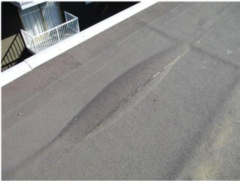
Another large blister near the roof perimeter.
