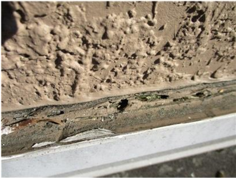
The sealant at the wall reglet or the top of counterflashing is missing or no longer functioning, possibly allowing water to channel behind the counterflashing.
