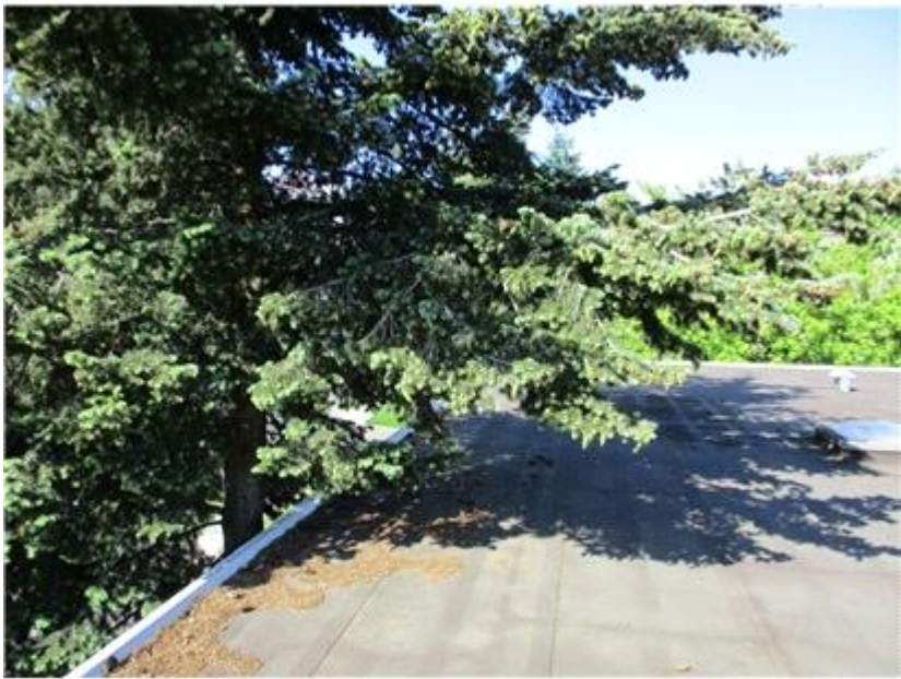
More overhanging trees depositing debris onto the roof.
