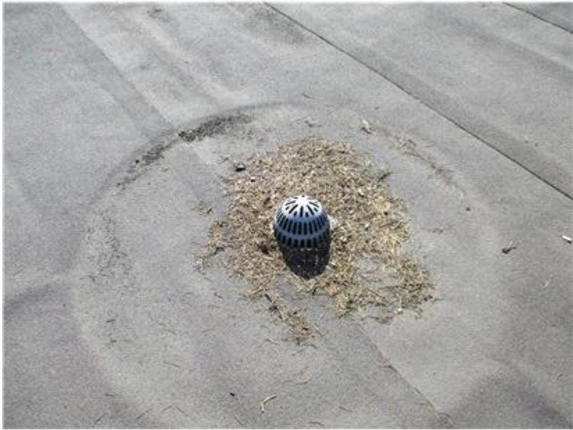
More debris blocking proper drainage at another roof drain.
