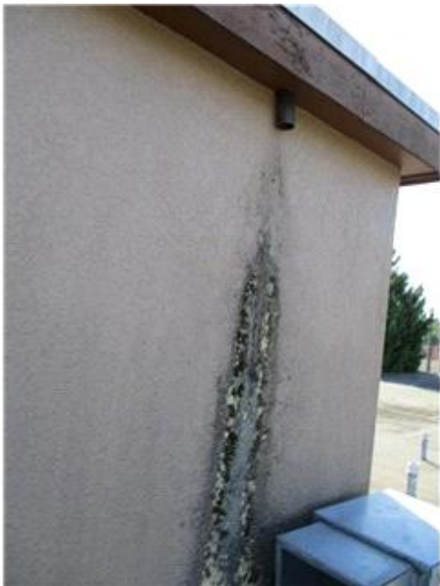
The downspout is missing from the scupper on this roof level. The draining water is staining the wall and may cause premature membrane erosion on the lower roof level.
