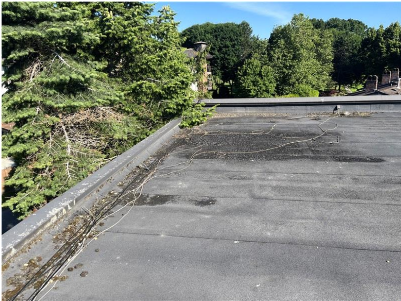
Overhanging trees were noted along the perimeter of this roof level.
