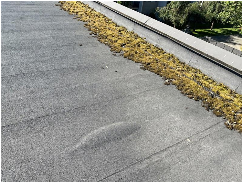
More organic debris and vegetation to be cleared off the roof surface.
