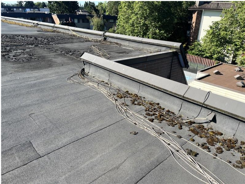
An accumulation of organic debris was noted on this roof level.
