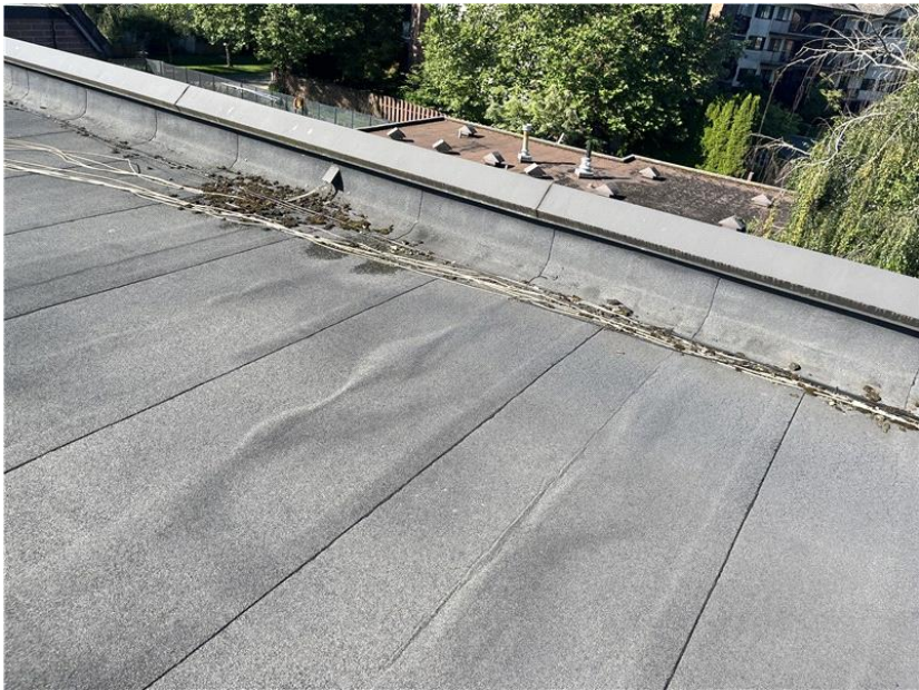
Another view of the cables directly on the membrane. More blisters and organic debris also noted.
