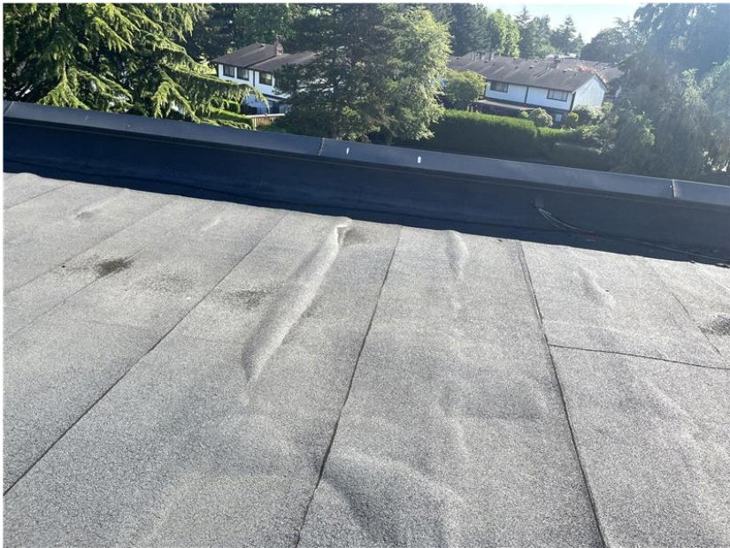
More blisters located in the field of the roof.
