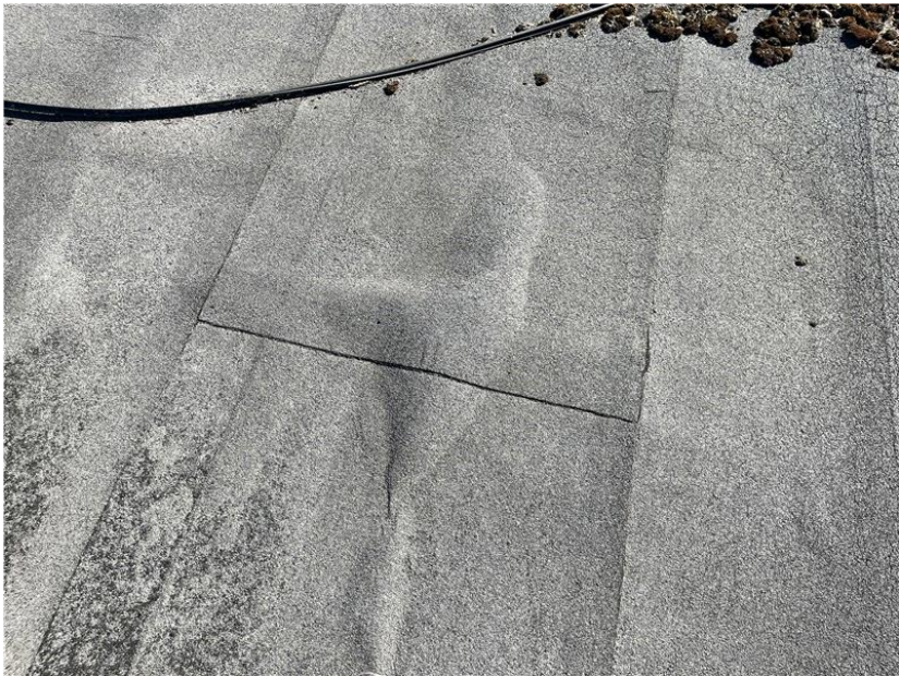
Another typical blister located in the field of the roof.
