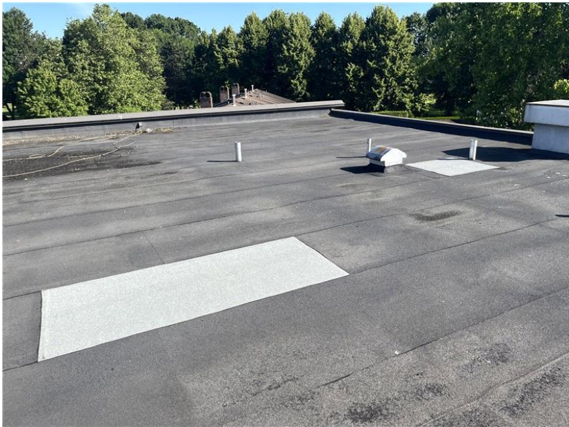
More modified bitumen membrane repairs completed previously.
