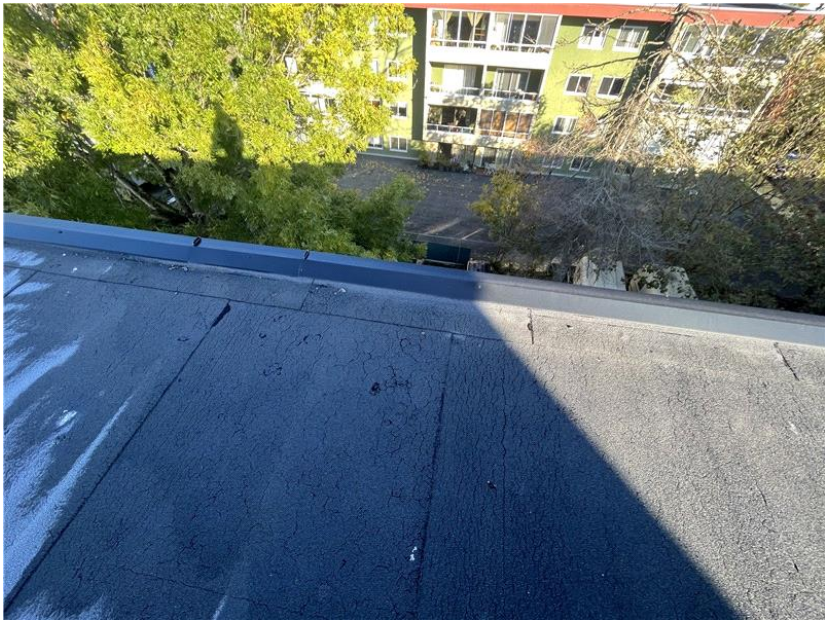
More damaged and cracked membrane.
