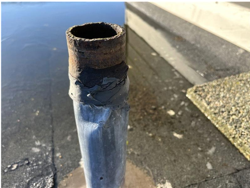
View of another corroded/damaged soil stack.
