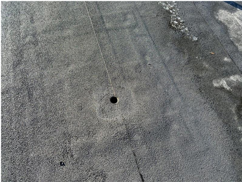
Another drain with missing drain guard.
