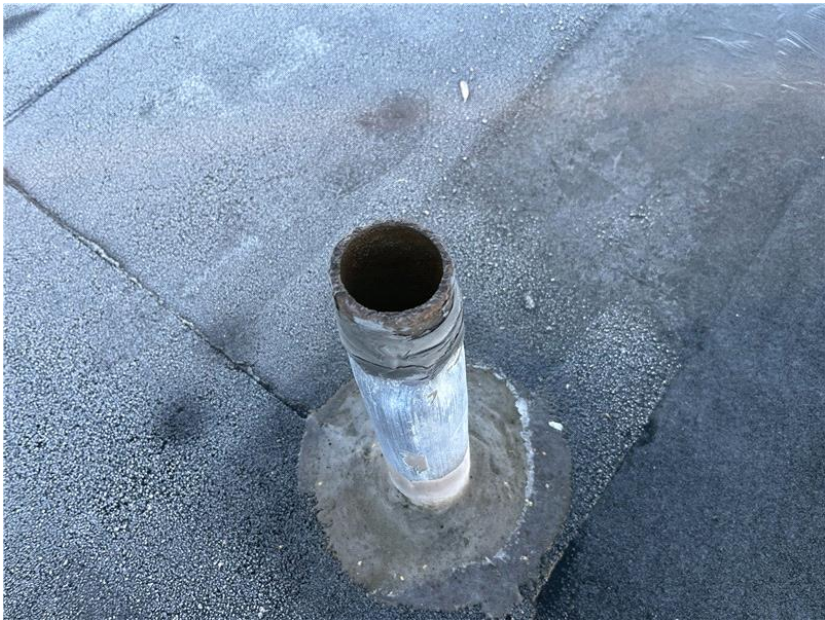
There is a missing stack cap around this soil stack. This condition may be allowing water to enter the roofing assembly and/or building.
