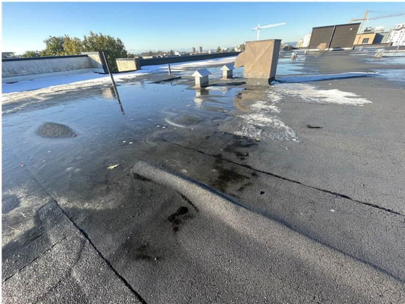
Another overview of the ridged and blistered membrane.
