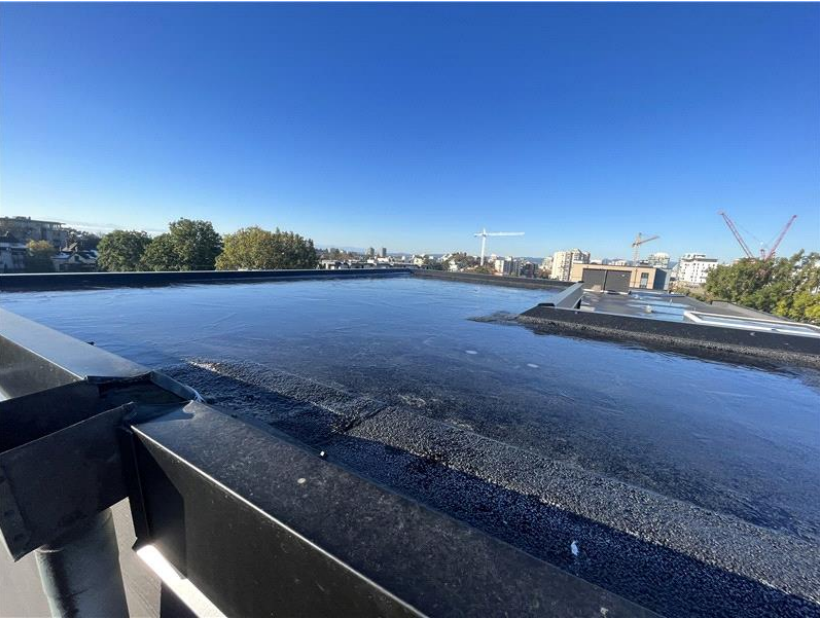
The roofing membrane is deteriorated with several under water blisters also noted.
