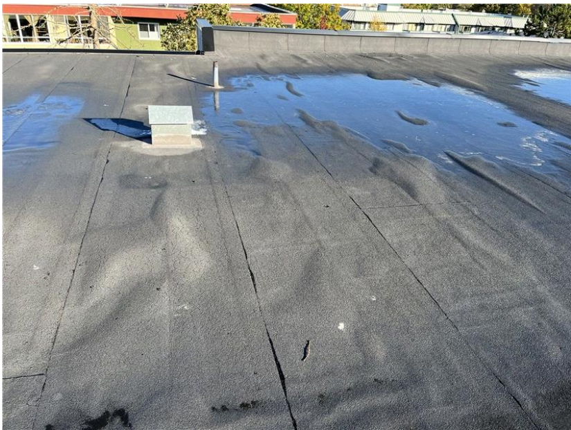
More blistered roofing membrane and areas with water ponding.
