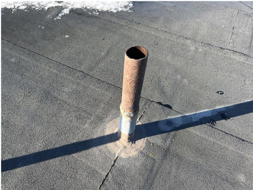
Several corroded soil stacks were noted on this roof level.
