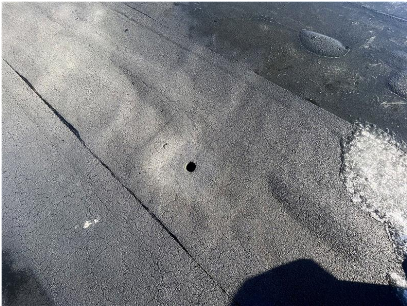
Another drain with missing drain guard.
