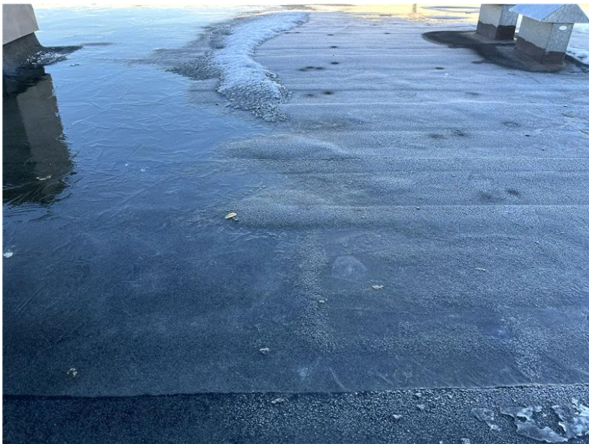
More blistered roofing membrane.
