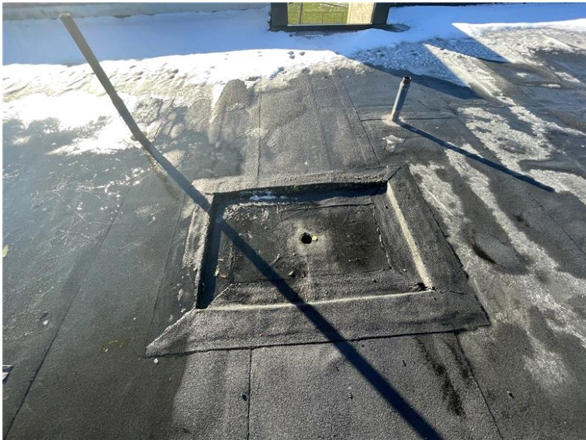
The drain strainer is missing. Without the screen in place, roofing debris may be able to enter the drainage system and impede proper water flow.
