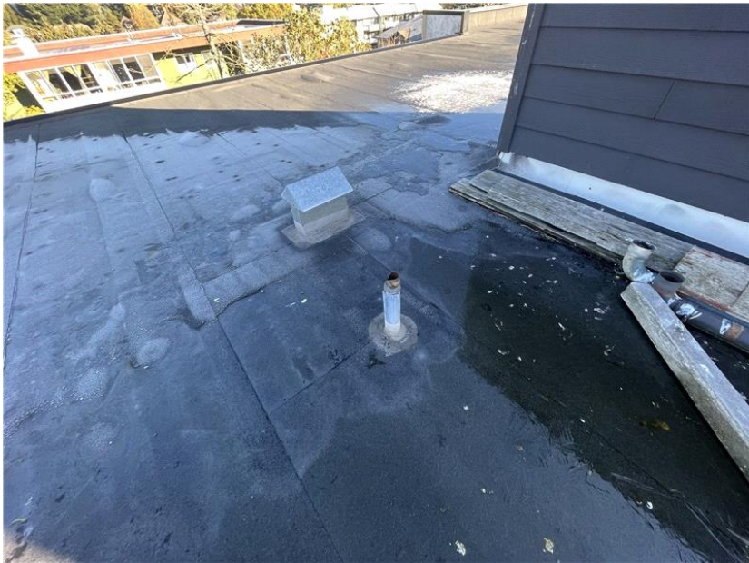
View of a corroded/damaged soil stack that was noted on this roof level.
