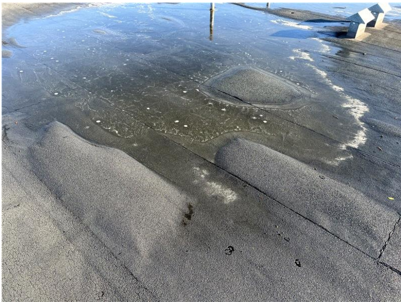
More blisters in the modified bitumen membrane.
