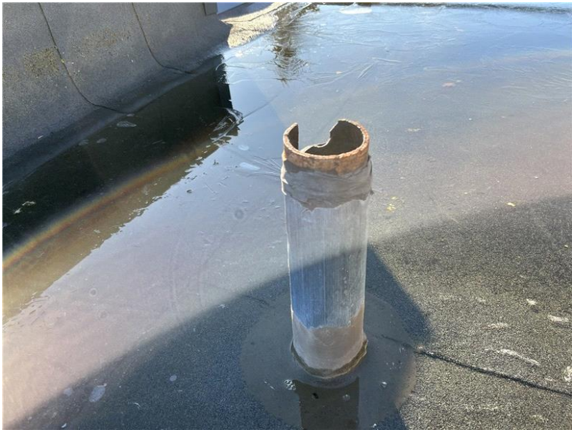
Another corroded/damaged soil stack.
