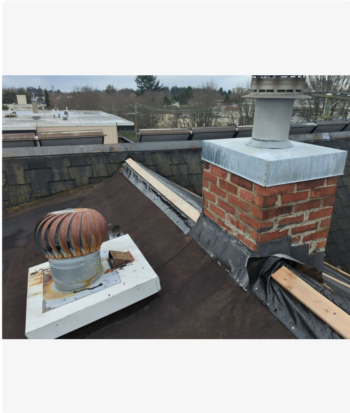
The chimney is in good condition.
