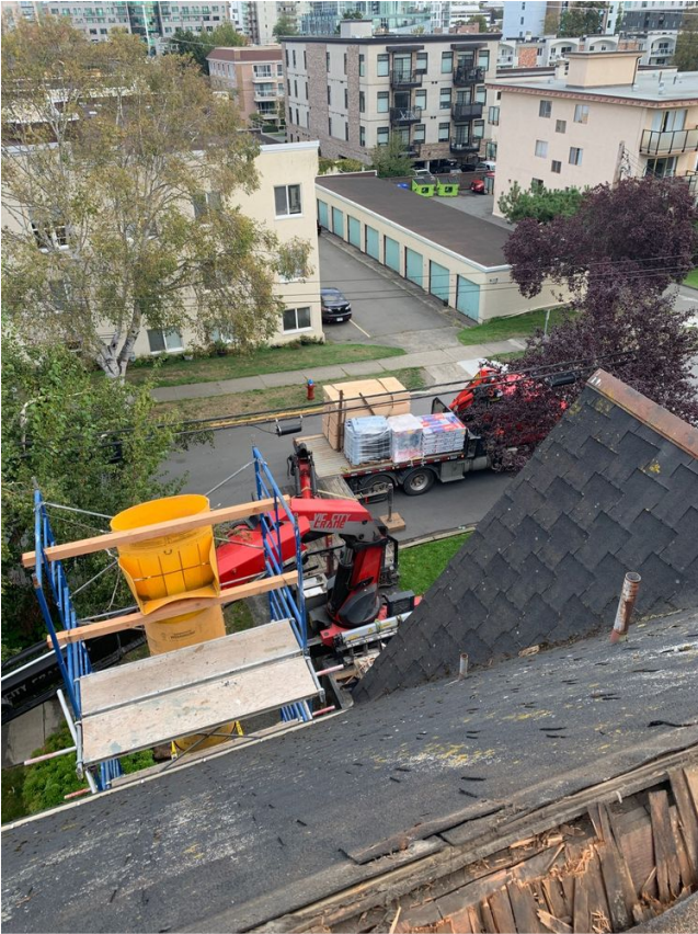
Garbage chute set up.
