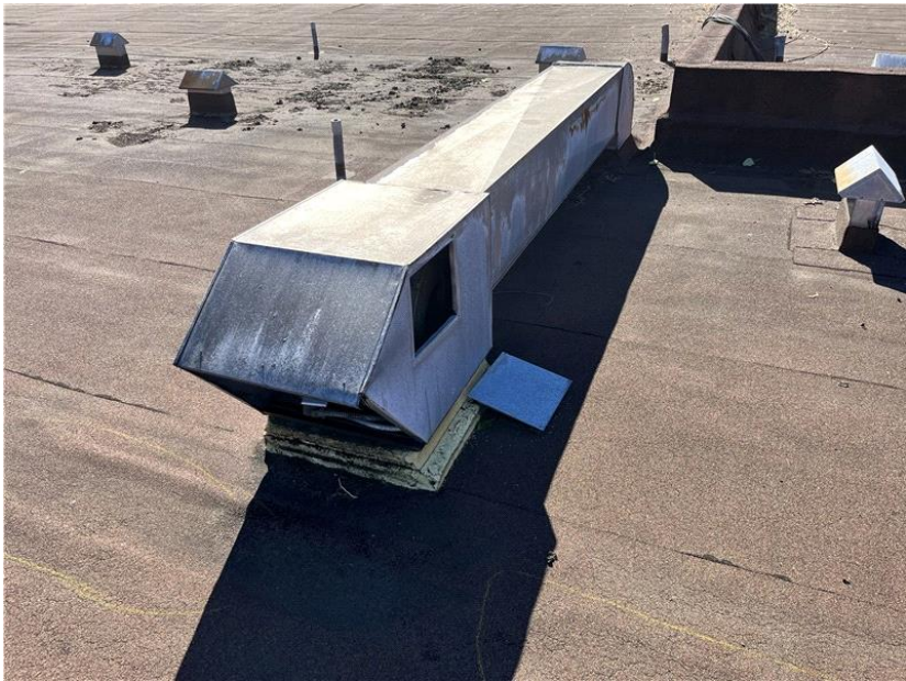
View of the unsecured access panel.
