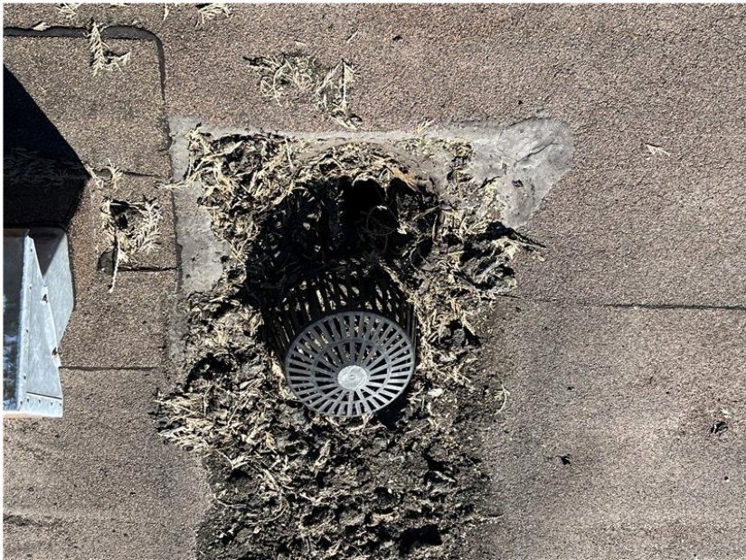
Close up of the organic debris around the roof drain.
