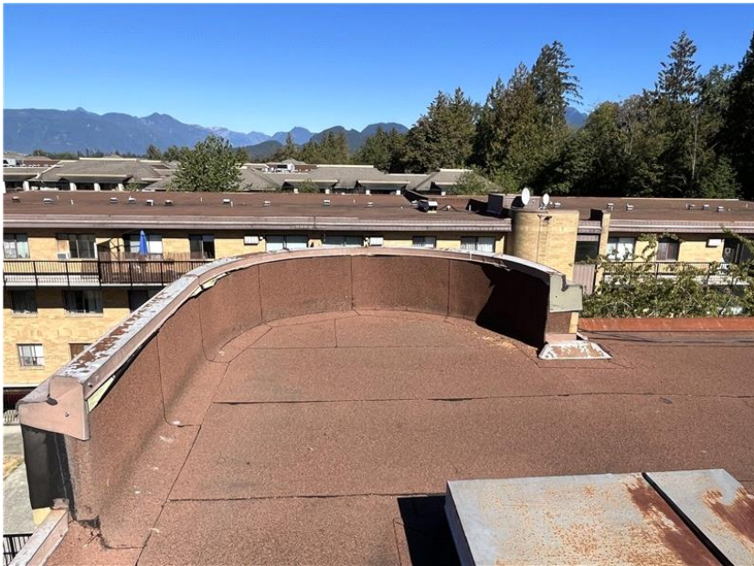
The perimeter metal flashings are corroded in several locations on this roof level.
