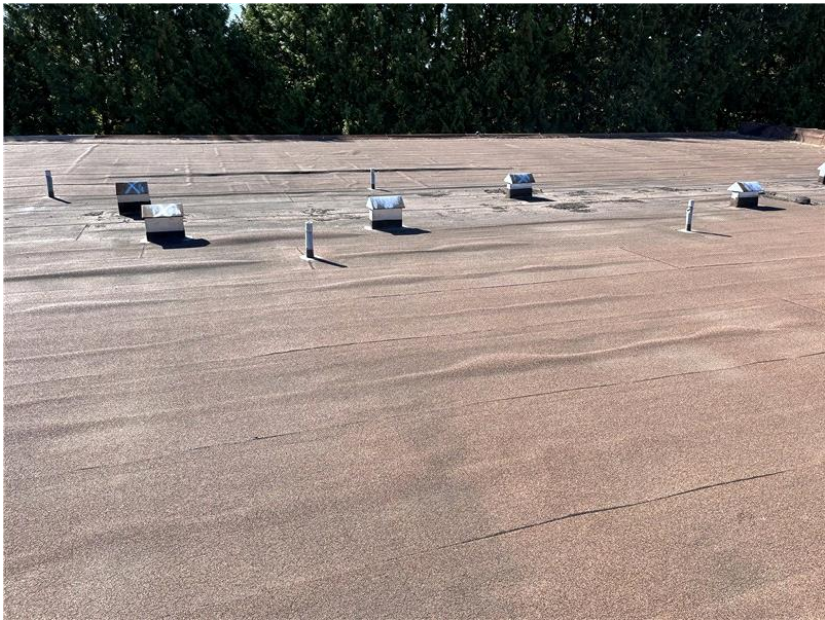
More blisters in the modified bitumen membrane.
