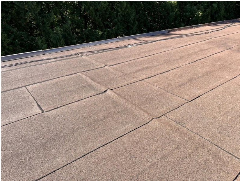
View of more wrinkles and ridges in the field membrane.
