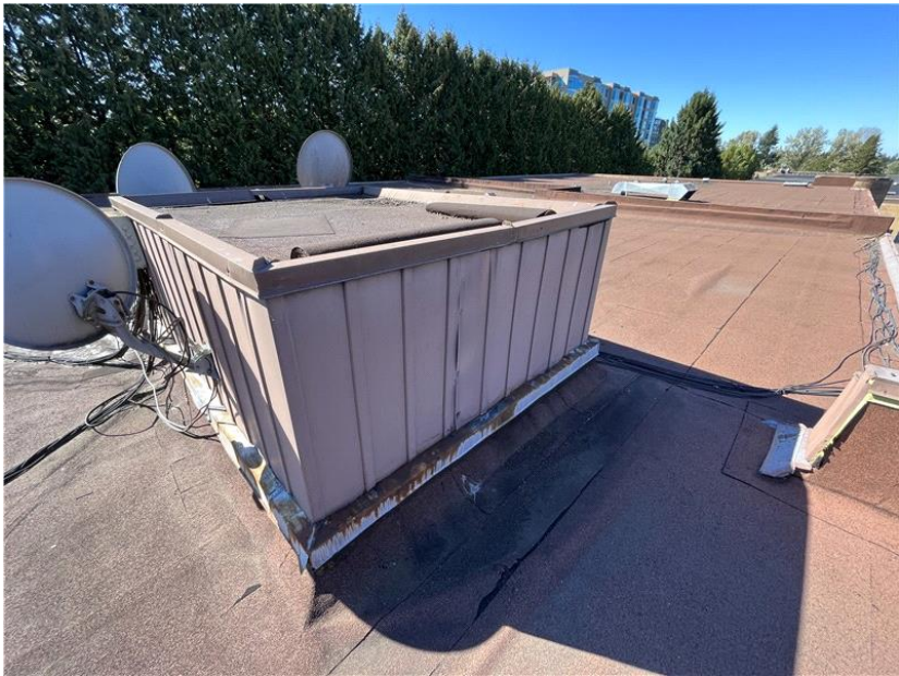
View of the severely corroded metal flashings on this roof.
