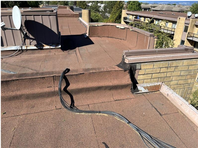
View of another previously completed temporary repair at the parapet.
