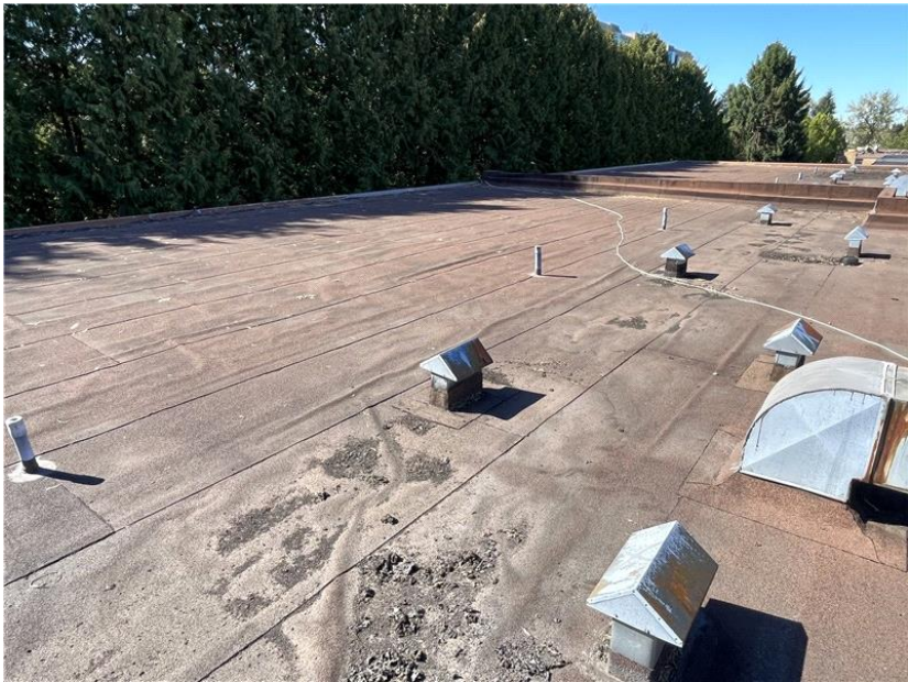
More blisters in the modified bitumen membrane.
