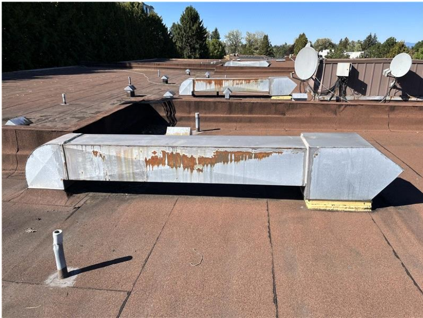
View of the corroded ductwork.
