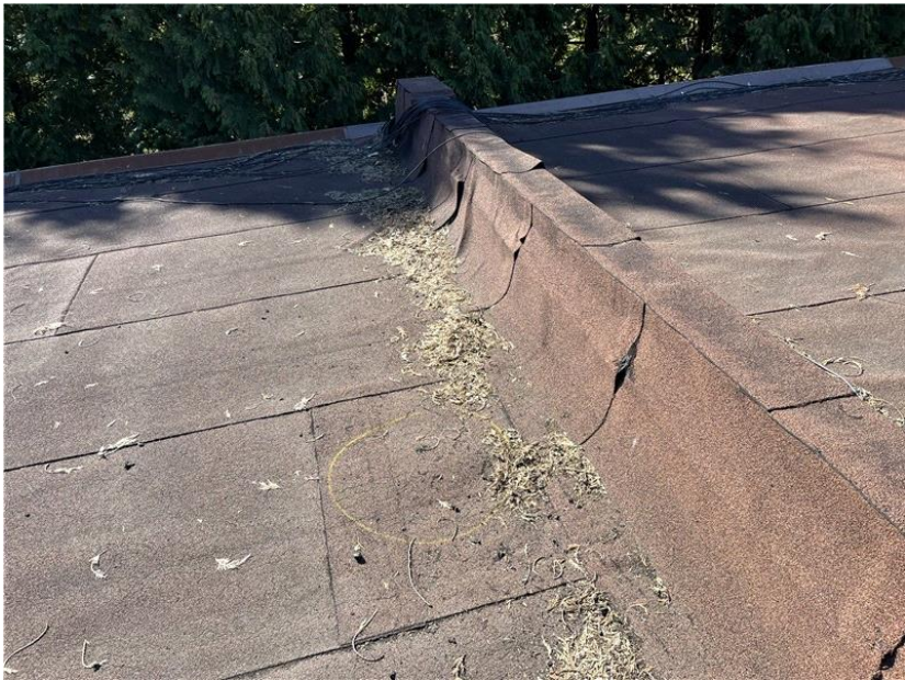
Another blister in the modified bitumen membrane.
