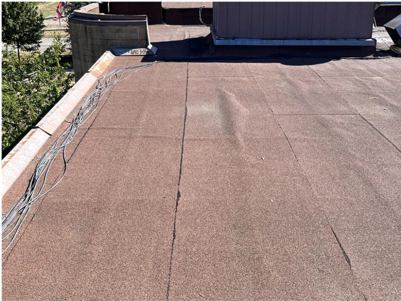
More blisters in the modified bitumen membrane.
