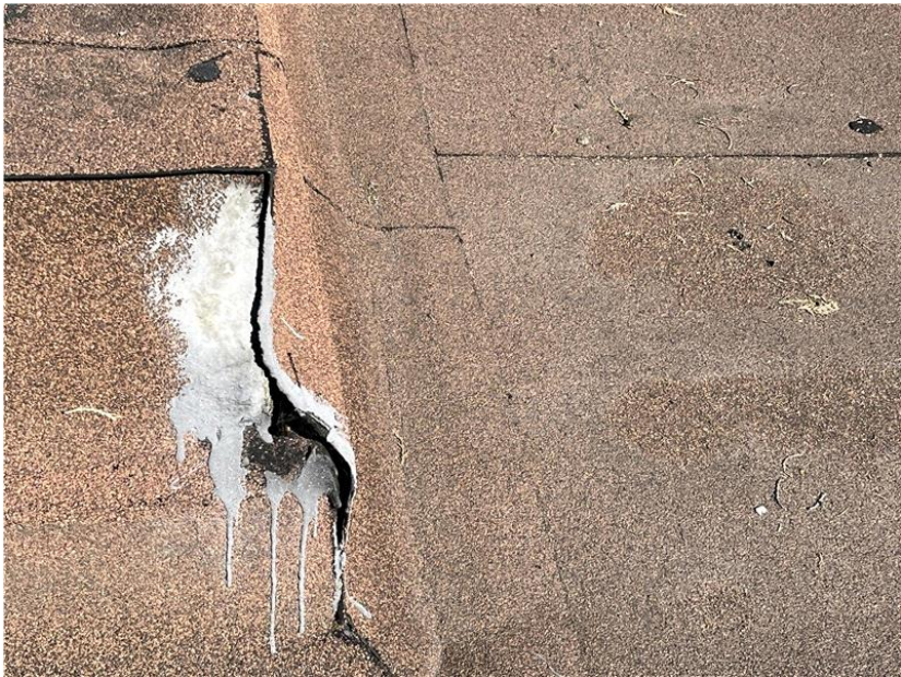
View of an improper repair in the field of this roof level.
