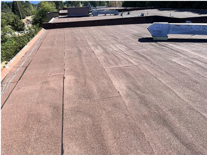
More blisters in the modified bitumen membrane.
