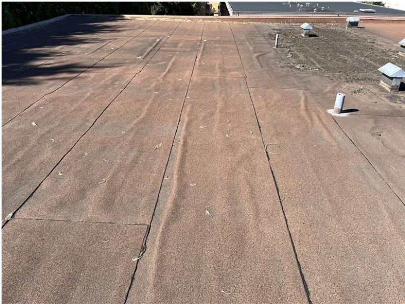
More blisters in the modified bitumen membrane.
