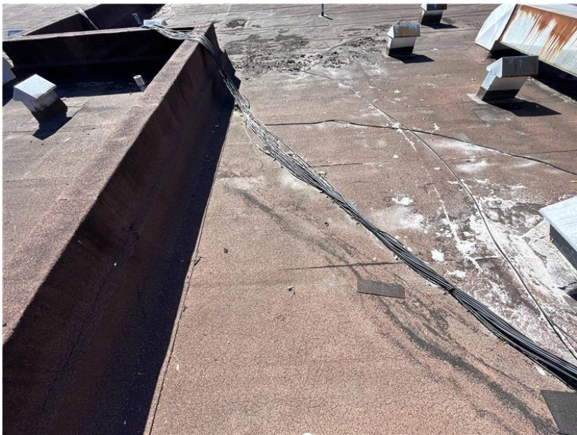
More improper/temporary repair in the field of this roof level.
