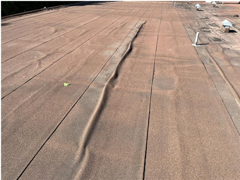
View of the wrinkles and ridges in the field membrane.
