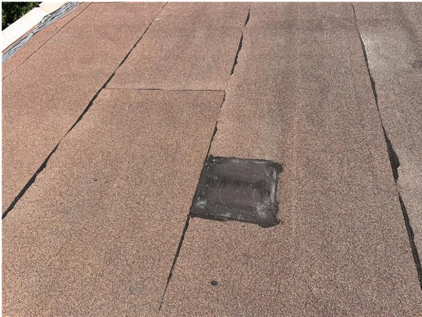
View of previously completed repair.
