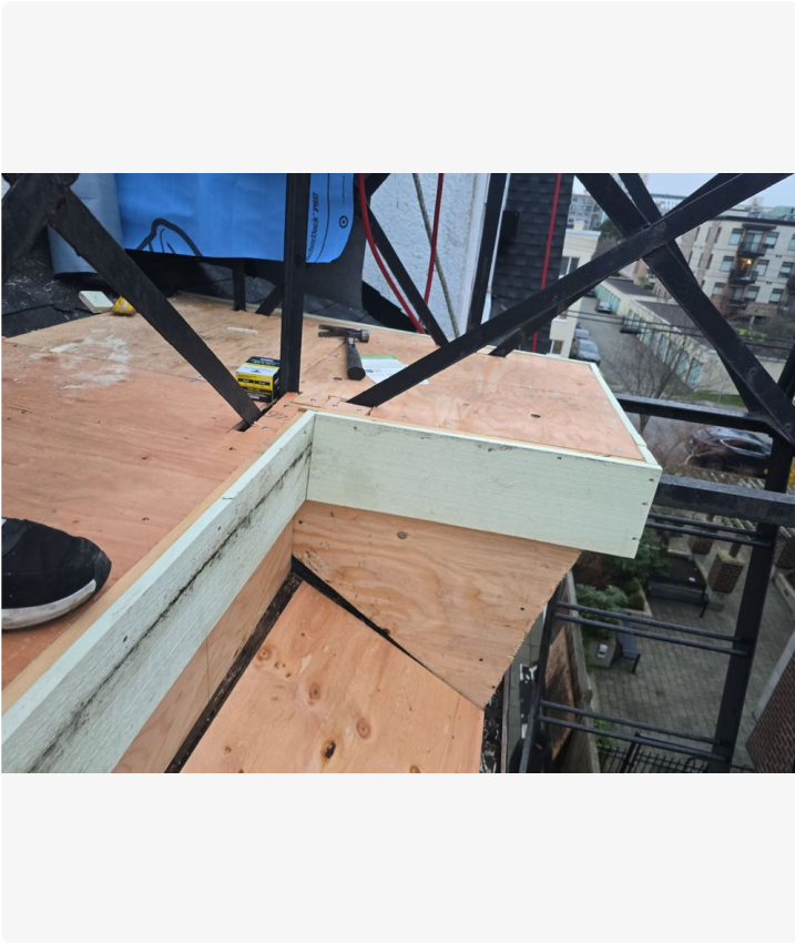
Project: Burdette Apartment Holdings Ltd. Date: Dec 4, 2024, 4:12 PM
