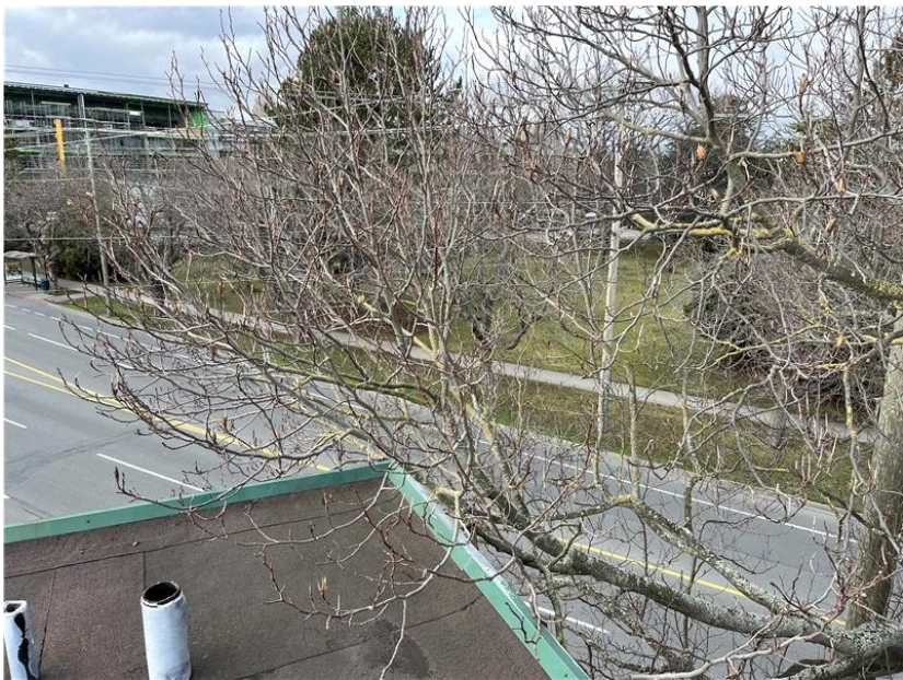
Overhanging trees were noted along the perimeter of this roof level. The tree branches may scrape the roofing membranes and and deposit organic debris onto the surface of the roof, which will clog roof drains and impede drainage.
