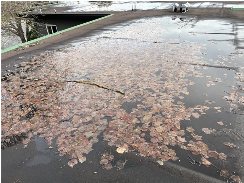
Large accumulation of organic debris was noted on this roof level.
