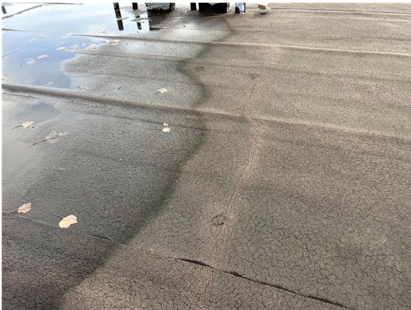
Another view of the alligatored roofing membrane.
