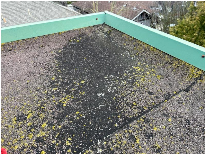
Another area with de-granulated cap sheet.
