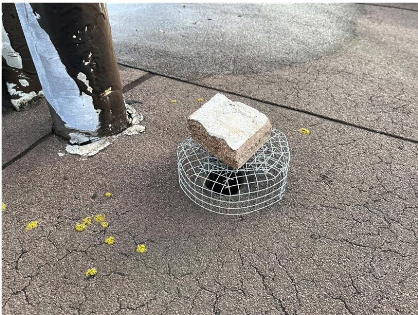
View of improper drain strainer held in place by a brick. Without proper screen in place, roofing debris may be able to enter the drainage system and impede proper water flow.
