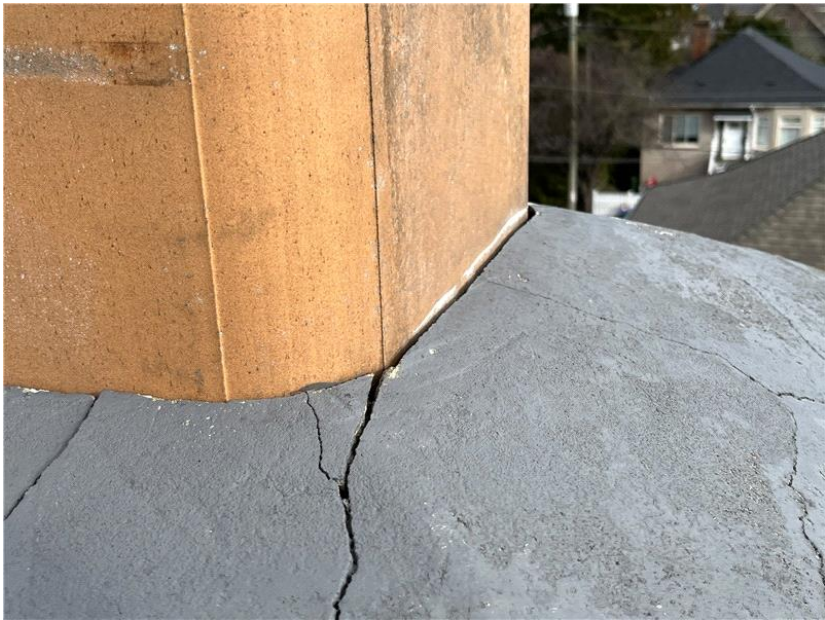
Close up of the cracks noted in the brick chimney.
