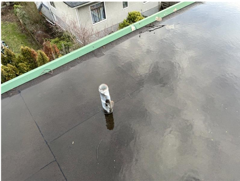
More ponding water and a damaged soil stack.
