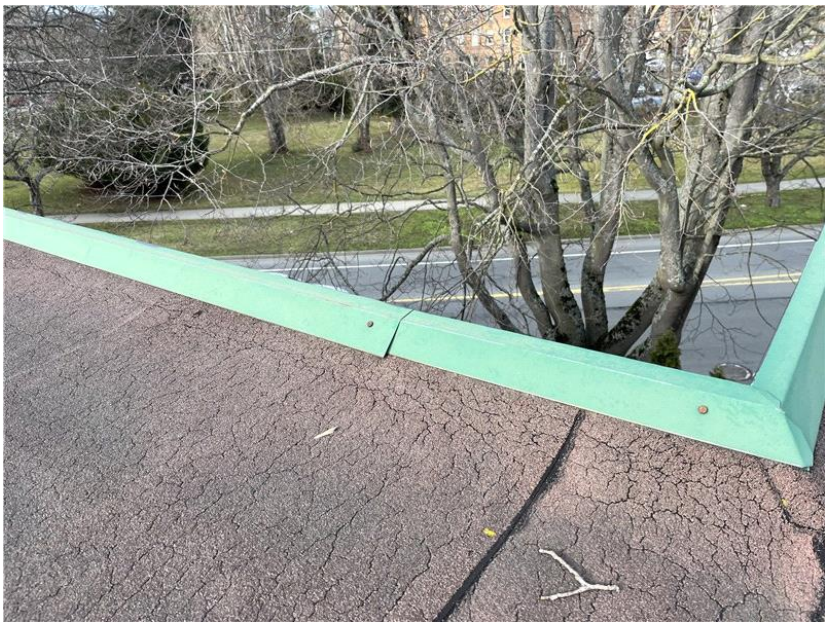
Metal cap flashings have been secured with standard roofing nails, which are also showing signs of corrosion. These sections are susceptible to leaks.
