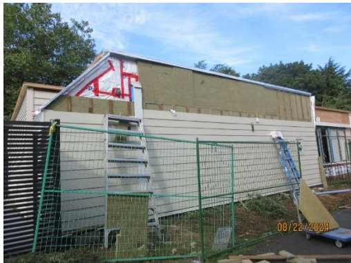
Photo 1): Ongoing siding installation on the east elevation.
