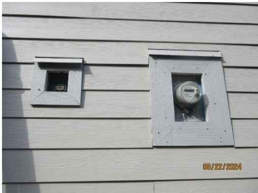
Photo 2): Trim and flashing at wall-mounted devices on the east elevation
