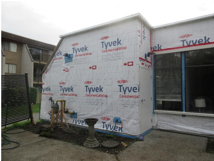
Photo 1): Siding installation in progress on the north elevation.
