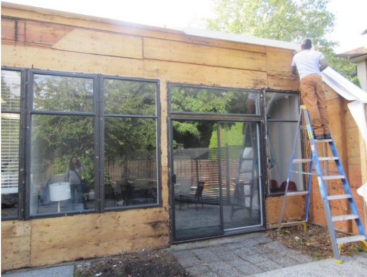
Photo 1): Demolition in progress on the north elevation.
