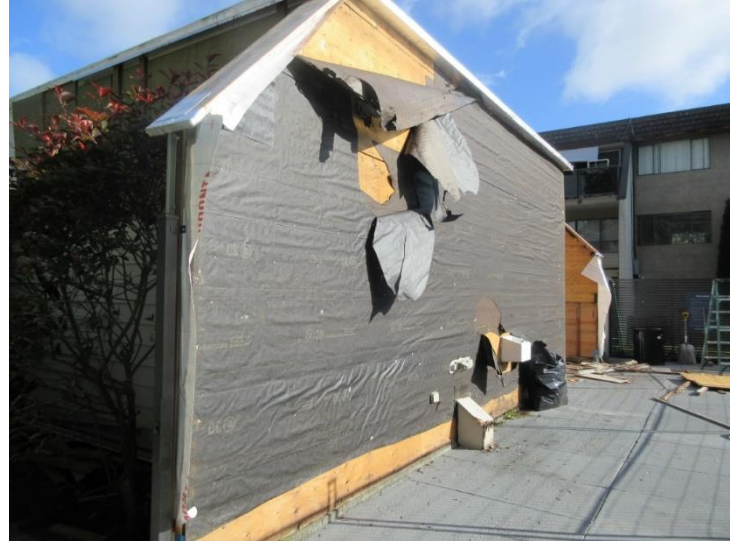
Photo 2): Demolition in progress on the south elevation.
