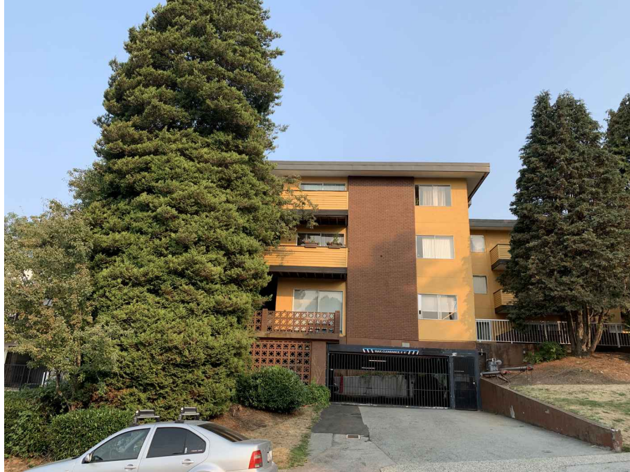
South side of the property.
