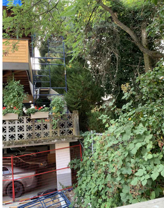
Example of metal scaffolds installed on the podium on the west side of the building for carrying out the proposed works
