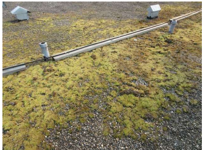
Photo 14: Typical original roof with extensive vegetation.
