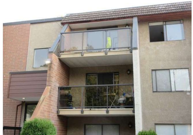
Photo 7: Typical exterior walls.
