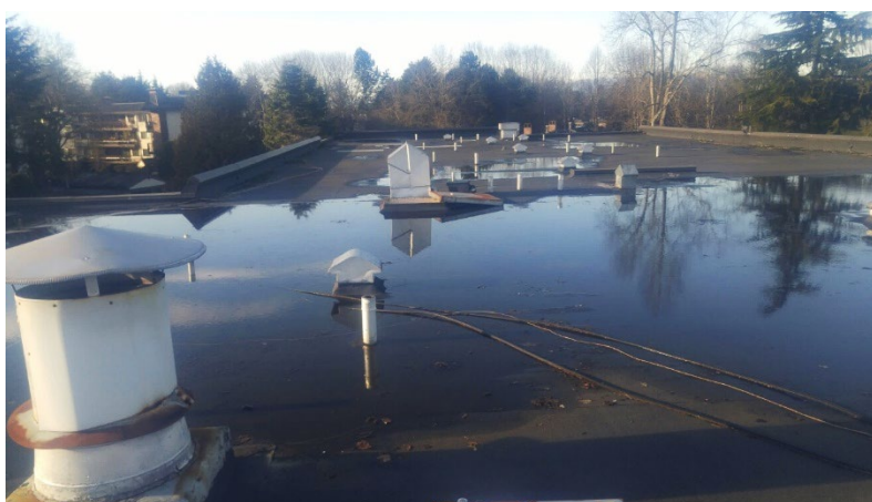
Photos 1 & 2 – Roof at 10851 Mortfield Road
