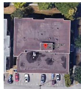
Figure 2 – View of Roof
